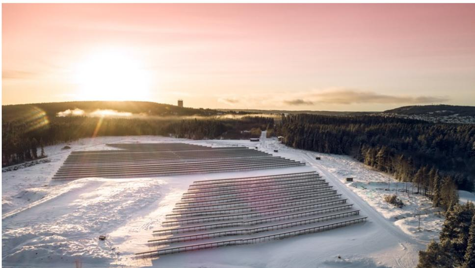
**Figure 6.4:** Östersund solar park. 10 000 panels with 3 MW peak power.[88]
